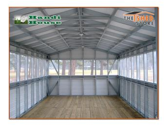
Our screen rooms are standard with steel studs, no windows, screen door. The number of lights and receptacles depends on the size of the unit ordered. Screen rooms also have a treated plywood floor or treated 2x6 lumber if requested for an additional cost.
